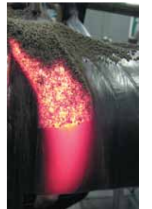
Corresist Submerged arc welding
