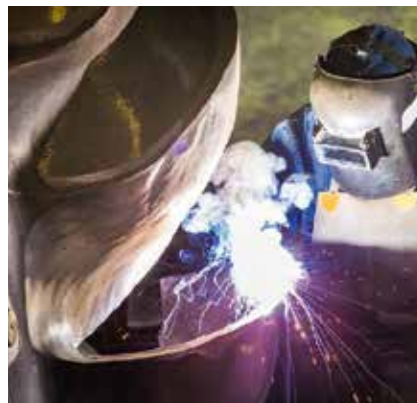
CHROMECORE B 13 4-G, repair of hydro Pelton bucket
