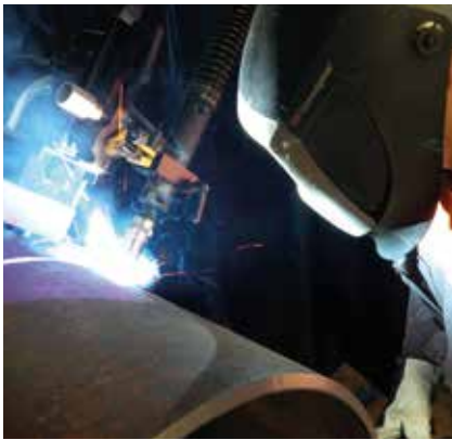
ROBOFIL M 700, pipe butt welding root to cap
