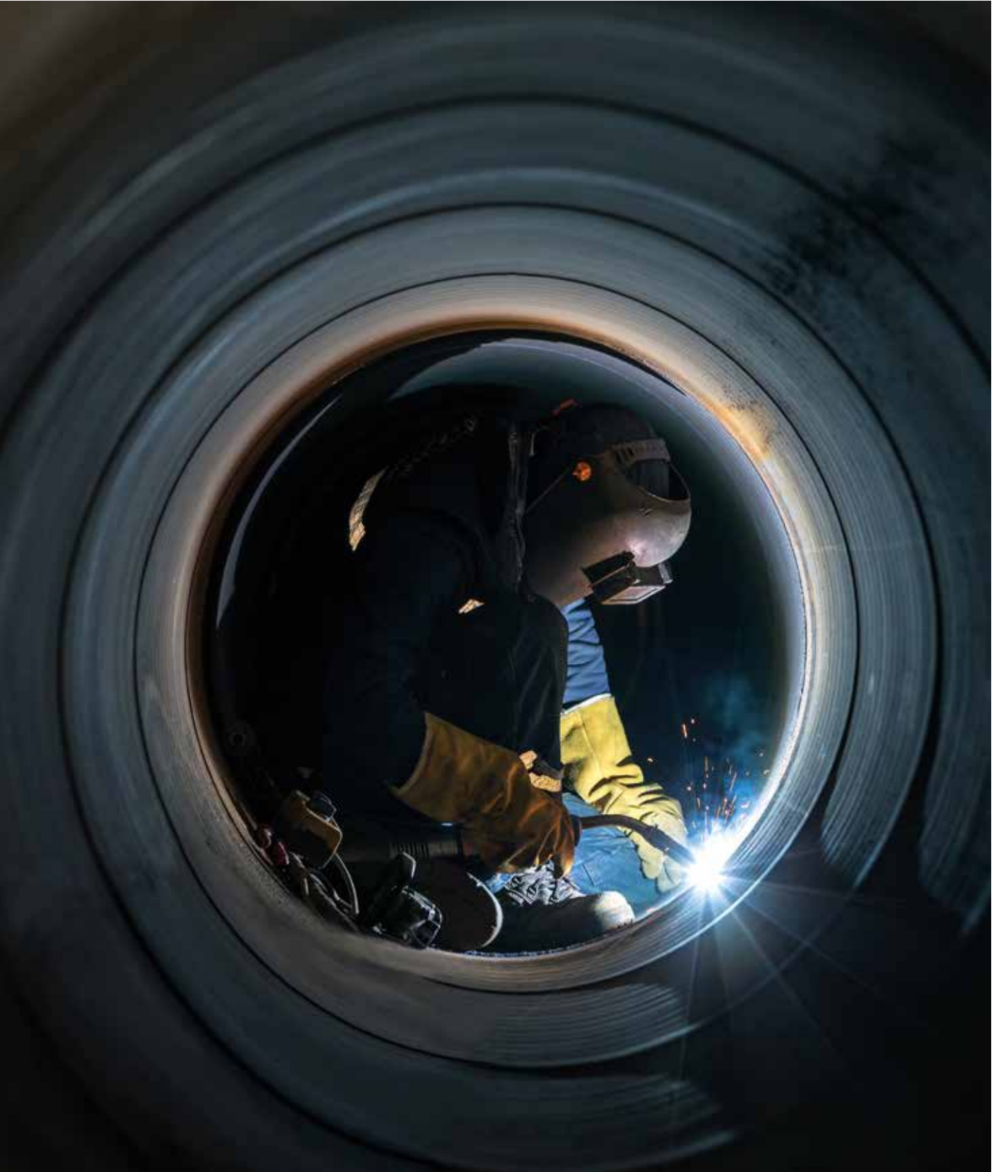
Back side welding of a V-groove joint using ROBOFIL M 71.
