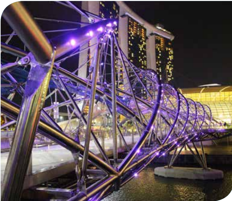
The Helix Bridge, Singapore - made of duplex stainless steel
