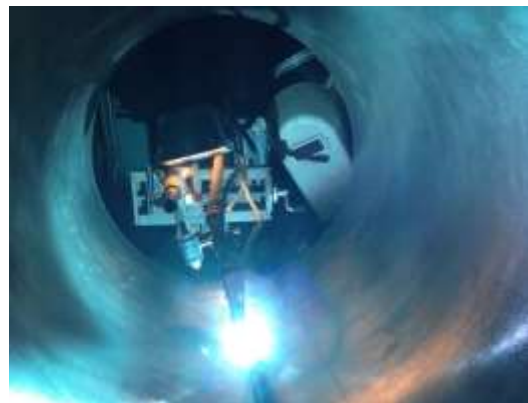
Figure 10 Longitudinal clad restoration GAMMA V 625
