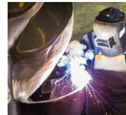
CHROMECore B 13 4-G, repair of hydro Pelton bucket
