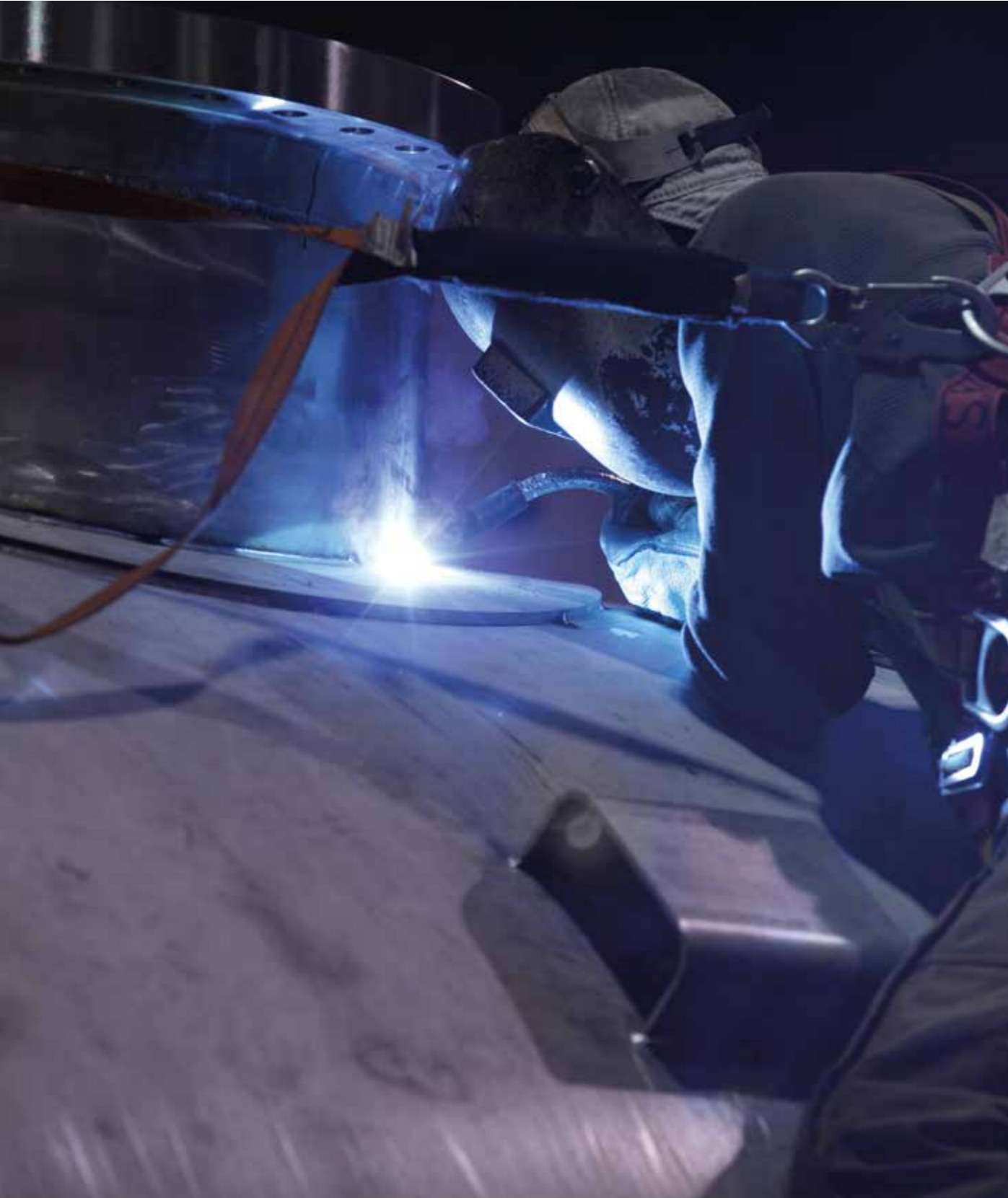
Joining of a reinforcing pad using our TETRA wire range.
